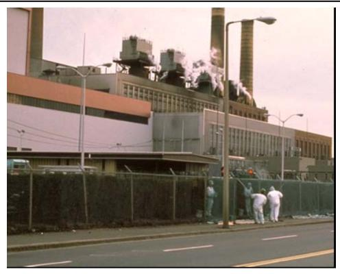
Painting crew at a major New England power station applies Endcor 4930 Series urethane primer-maintenance coating from Dampney Company Inc. to protect and improve the appearance of perimeter fencing. A single coat of the flexible, impact-resistant coating protects even marginally prepared rusted surfaces from corrosive salt air and industrial environments. Endcor 4930 cures under highly humid conditions in temperatures as low as 10°F (12°C).
